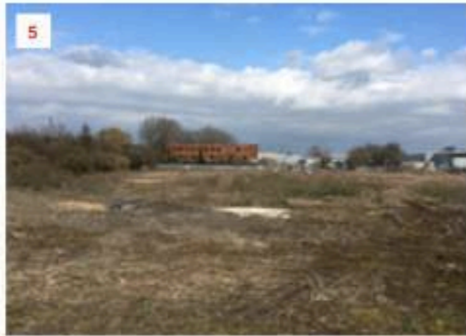
View of Northern Site looking east
