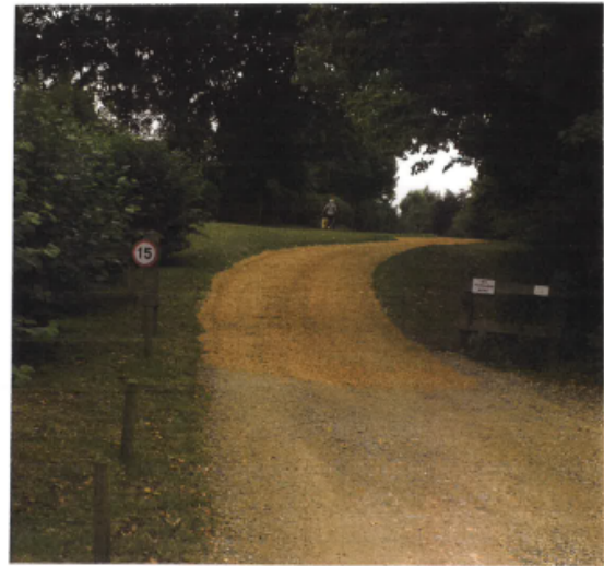
APPROX 3.0M SLOPE FROM THE FARM UP TO THE MAIN GREEN. AT \pm 72.00
